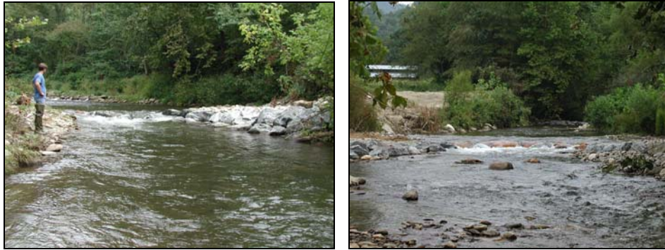
J-Hook and cross vane structures on Soco Creek
