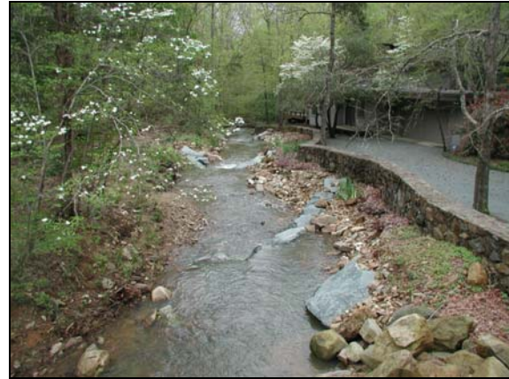
Cedar Branch 2 years after construction. The cross vanes are used to reduce stress next to the rock wall and dissipate energy through a step pool channel
