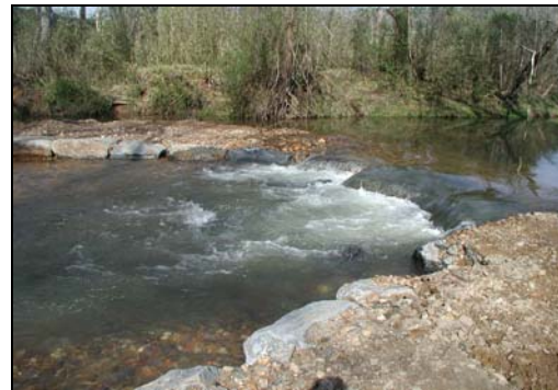
In-stream structures were placed in the channel to improve habitat and protect streambanks
