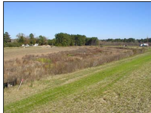
Restored channel with floodplain construction
